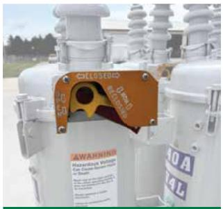
An oil circuit recloser, like you see here, helps protect the electric system from a momentary power disruption when a bird, critter, or tree branch makes contact with the energized power line.
