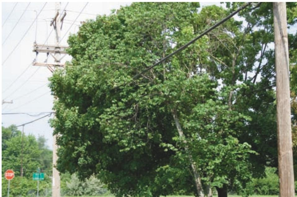
National standards for electrical safety require that branches within 15 feet of electrical equipment be removed. Be careful when trimming tree branches near power lines. If a tree presents a safety concern call the cooperative for help.
