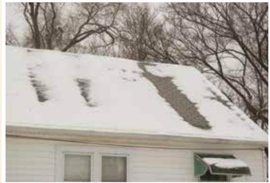
*Are your shingles shimmering with frost? Great! Frost (or the lack thereof) can be an indicator of how attic insulation is performing. Bare spots may mean insulation has fallen or holes/gaps exist. Even small gaps in the insulation can create space for heat to escape out your roof. Check your roof the next time there is adequate frost or light snow on it.*
